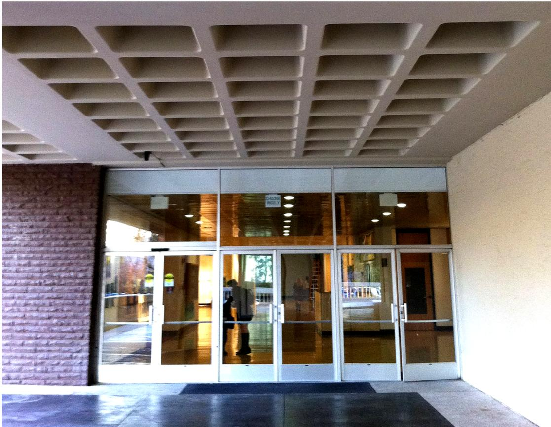
FIGURE 5.3: Waffle ceiling above the doors to the main entrance
