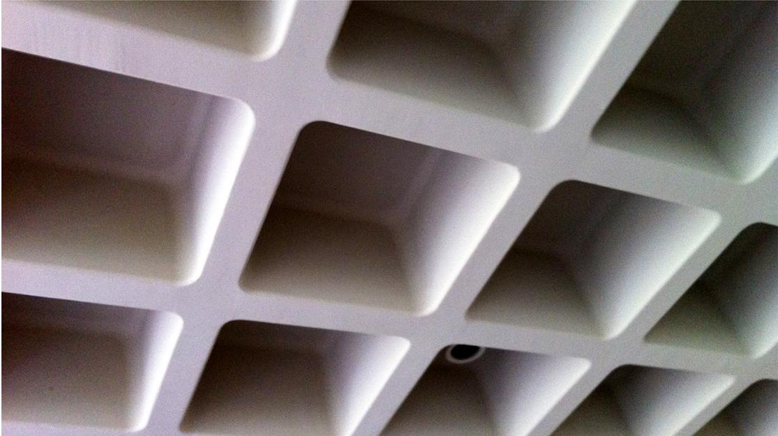
FIGURE 5.6: A detail view of the waffles. Mmm, waffles.
